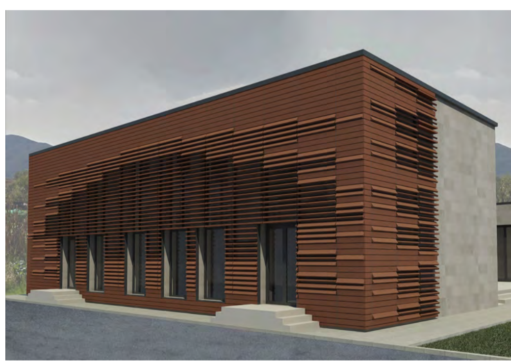
Renovation project and new construction Primary school San Donato, Lucca (Designed by P. Artini, V. Brogi, A. Pucci)
